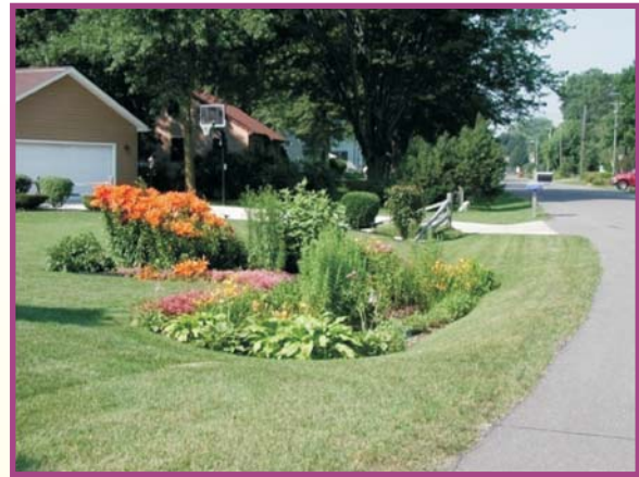
A soil storage and rainwater seepage system
