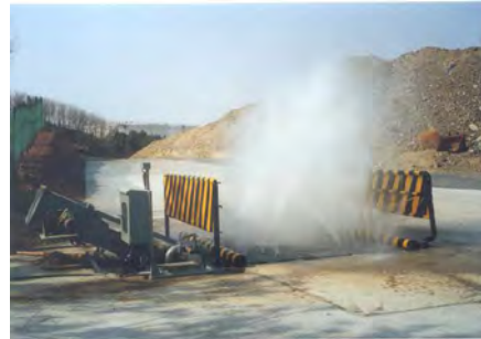
Fig. Annex- 34 Automatic washing system
