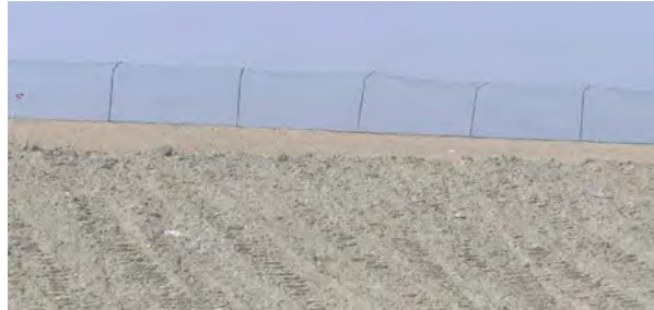
Fig. Annex- 33 Facilities to prevent scattering
